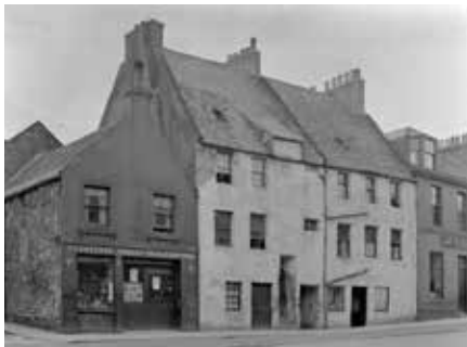
249-255 High Street (to the west of New Well Wynd) before demolition.
