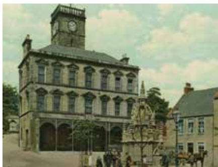
The metal piazza and sloping roof of the Burgh Halls.
