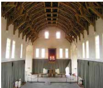
The timber roof in Stirling Castle banqueting hall.
