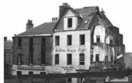
The Golden Cross being demolished.
