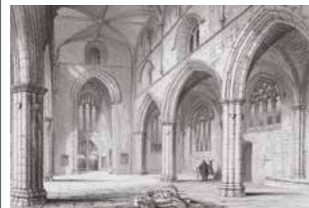
St Michael's in need of repair.
