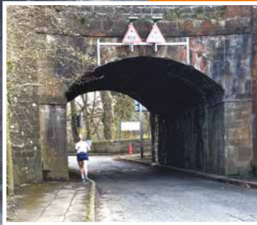
“CHOKE POINT AT CANAL BRIDGE”
